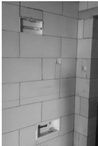
图2 “砖包管”施工工艺
